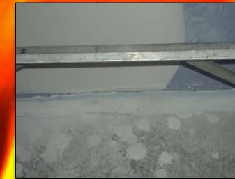
Bottom of Wall
