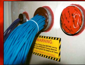
Tele-Data/Electrical Penetrations
